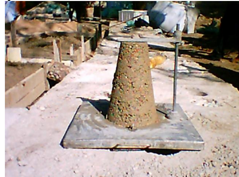
Fig. 10: Verification of no slump
