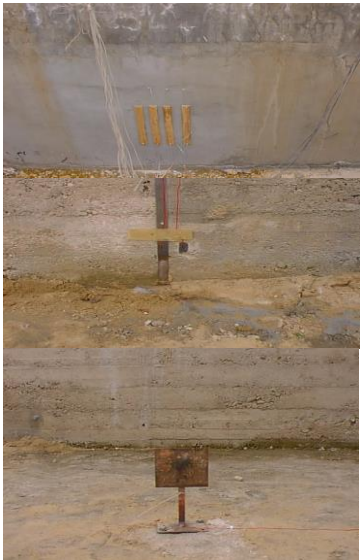
Fig. 24: Installing piezometers, electrical strain gauges, and pressure cell
