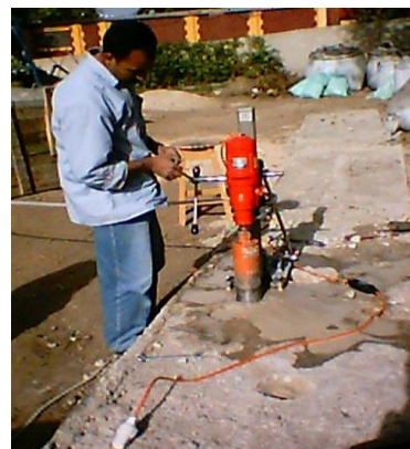
Fig. 13: Drilling concrete core machine
