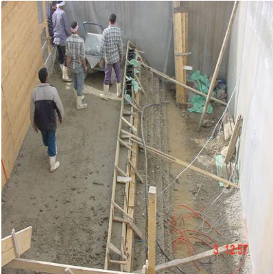
Fig. 20: Concrete placement into one of dam-layers
