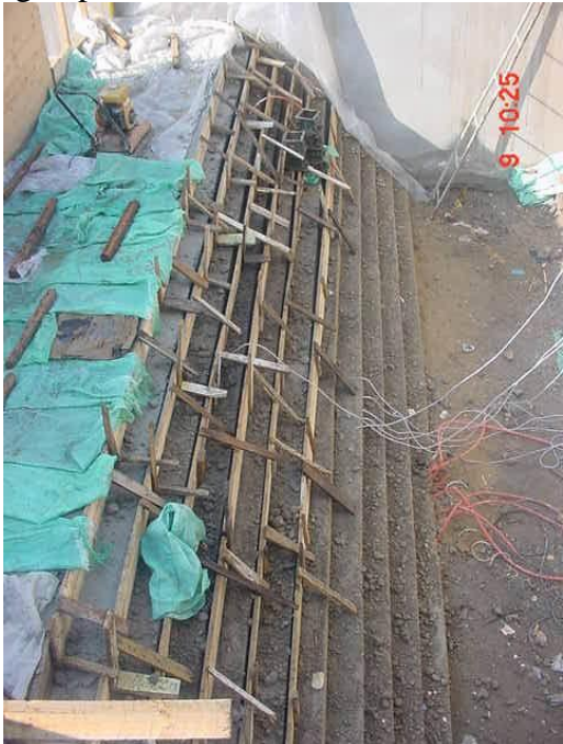
Fig. 23: Plastic covering for casted layers
