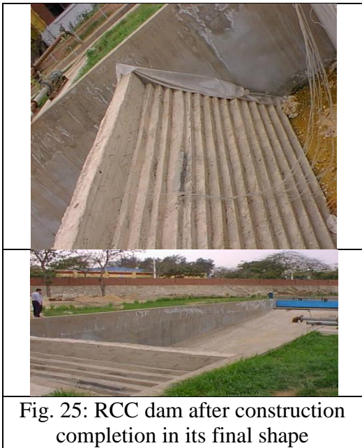
Fig. 23: Plastic covering for casted layers
