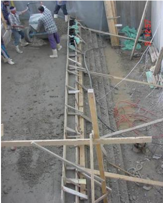
Fig. 19: Layering dam into 20 cm layers-thickness
