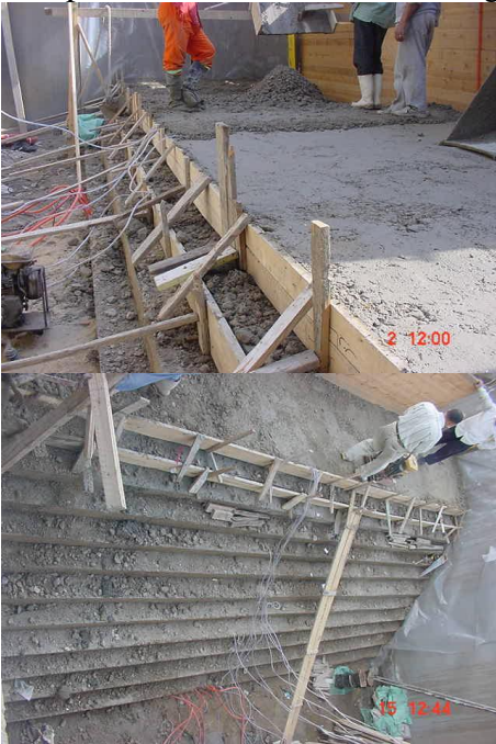
Fig. 22: Strengthen formwork during placement
