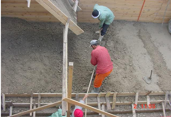
Fig. 18: Remixing the concrete manually
