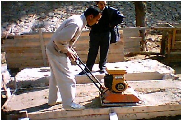
Fig. 9: Trial slabs compacted with soil compactor
