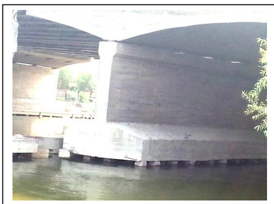
Photo (1): Mestored bridge at Cairo-Egypt
