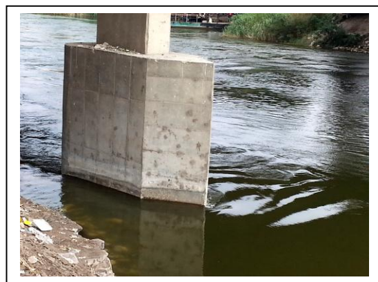
Photo (2) Mataria bridge at Cairo-Egypt
