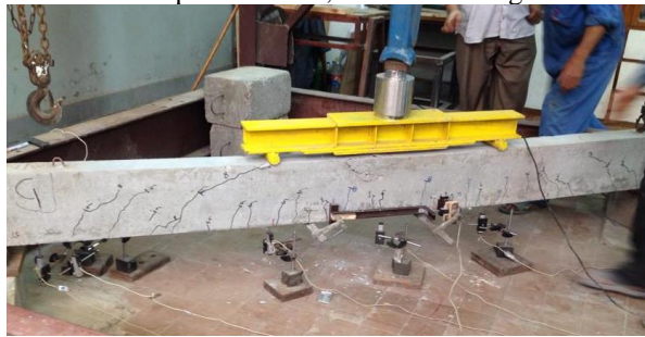
Fig.21: shows failure mode of un-wrapped (A1).
